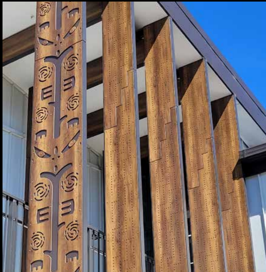
University of Otago - Dental Facility, Auckland Design, Supply and Installation 10mm Fundermax Routed Design Cladding
