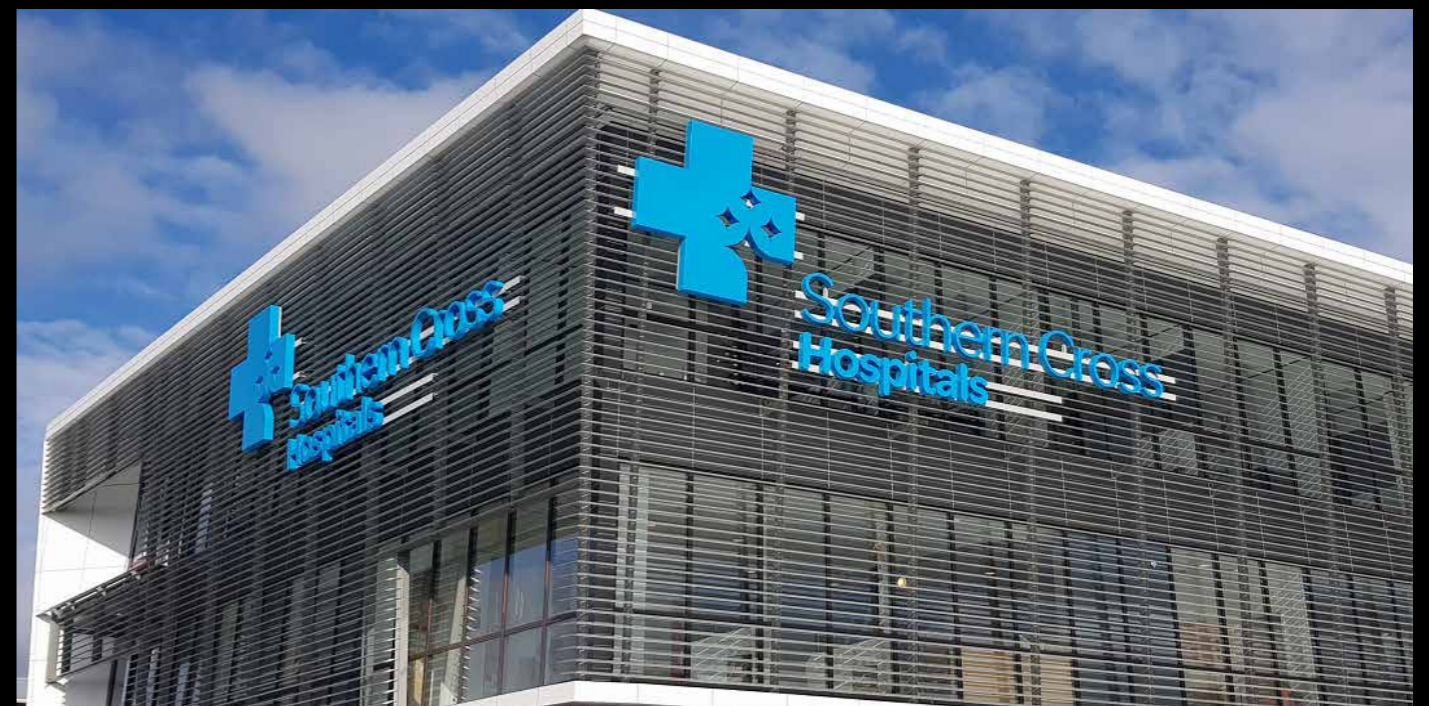
Southern Cross Hospital Northern Clinic, Auckland Design, Supply and Installation Aluminium Solar Shading and Support System
