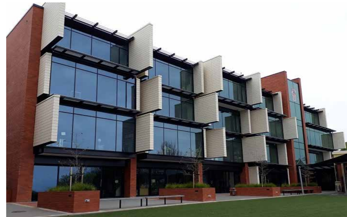
King's School, Auckland Design, Supply and Installation 30mm Thick Terracotta Tiles and Baguettes
