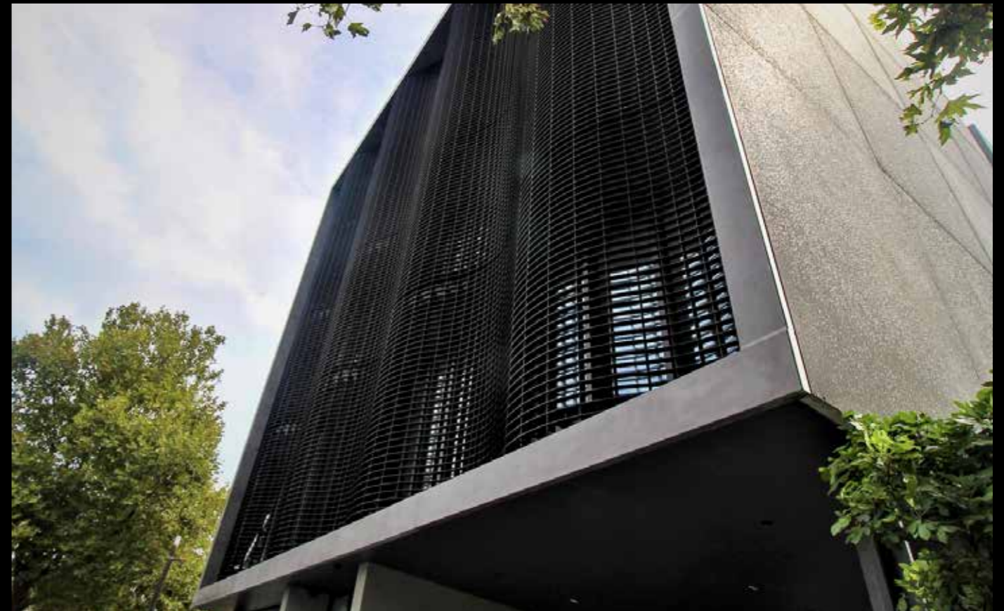
Jervois Road Apartments, Auckland Design, Supply and Installation 15mm Thick GRC Feature Cladding
